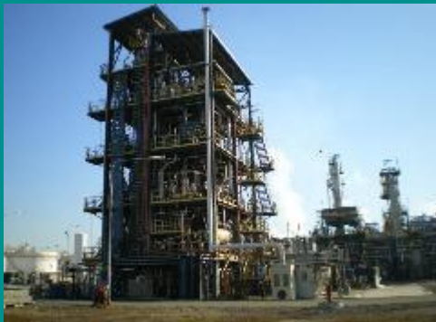
FT Demo Unit- Sanazzaro
