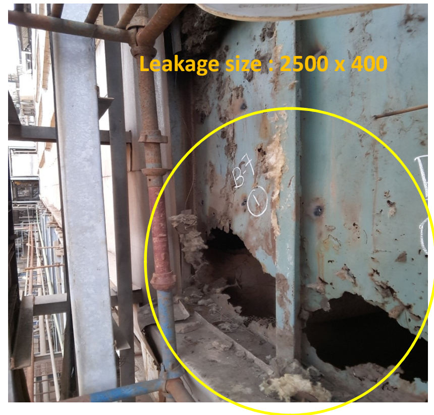
ESP SIDE CASING
