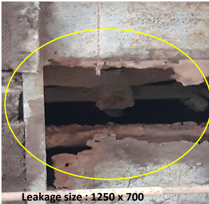
ESP SIDE CASING
