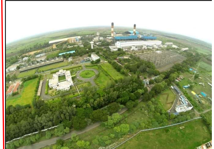
4x125 MW Lignite Based CFBC Units Phase-I (Year 2000), Phase II (Year 2010)
