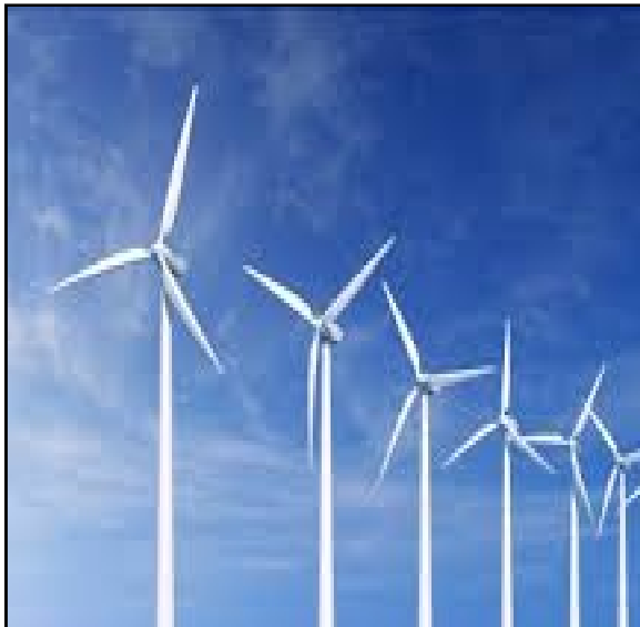
112.4 MW Wind Power (2017)
