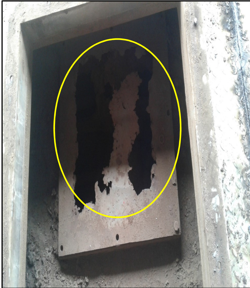
ESP INNER ROOF /MHD : BEFORE
