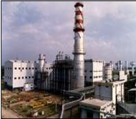
Gas Based Power Plant 145 MW (Year 1992) 165 MW (Year 1997)
