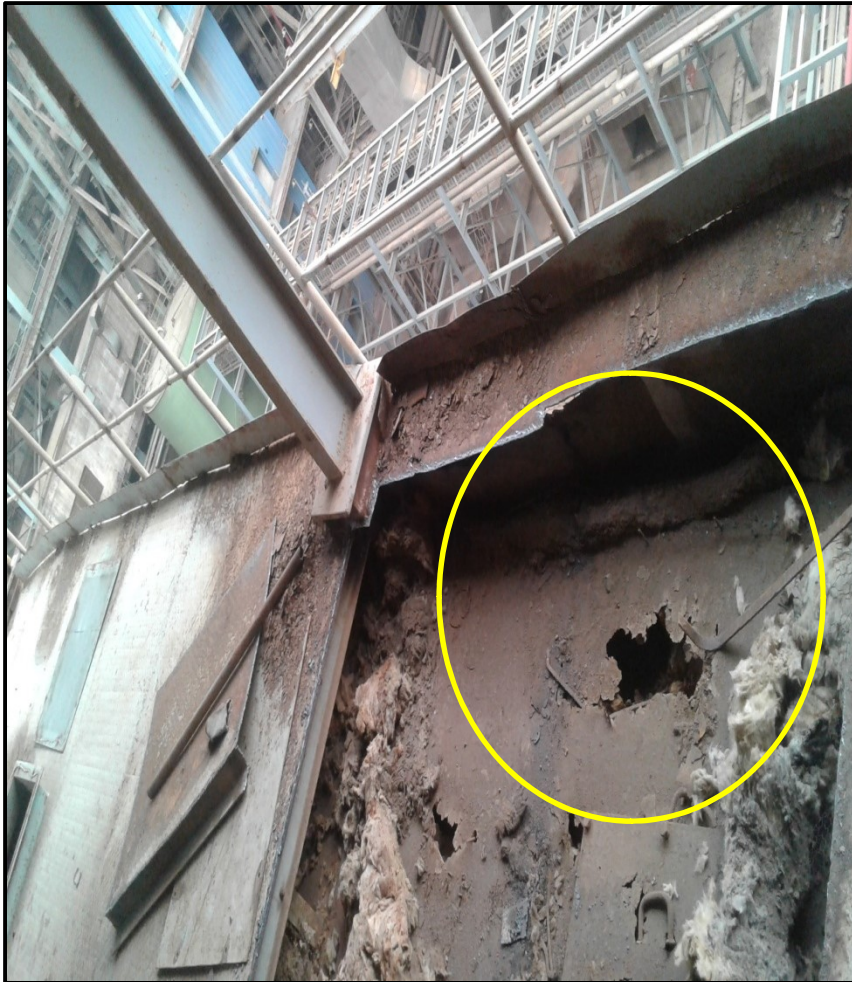
ESP INNER ROOF CASING PLATE : BEFORE
