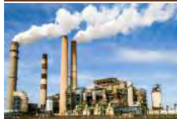
Power Plant Performer ≥ 500 MW – CCGT
