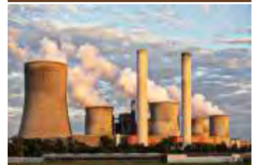
Power Plant Performer – CCGT (CPP)
