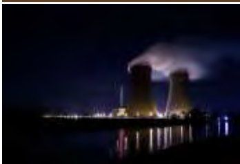
Power Plant Performer ≤ 500 MW – CCGT
