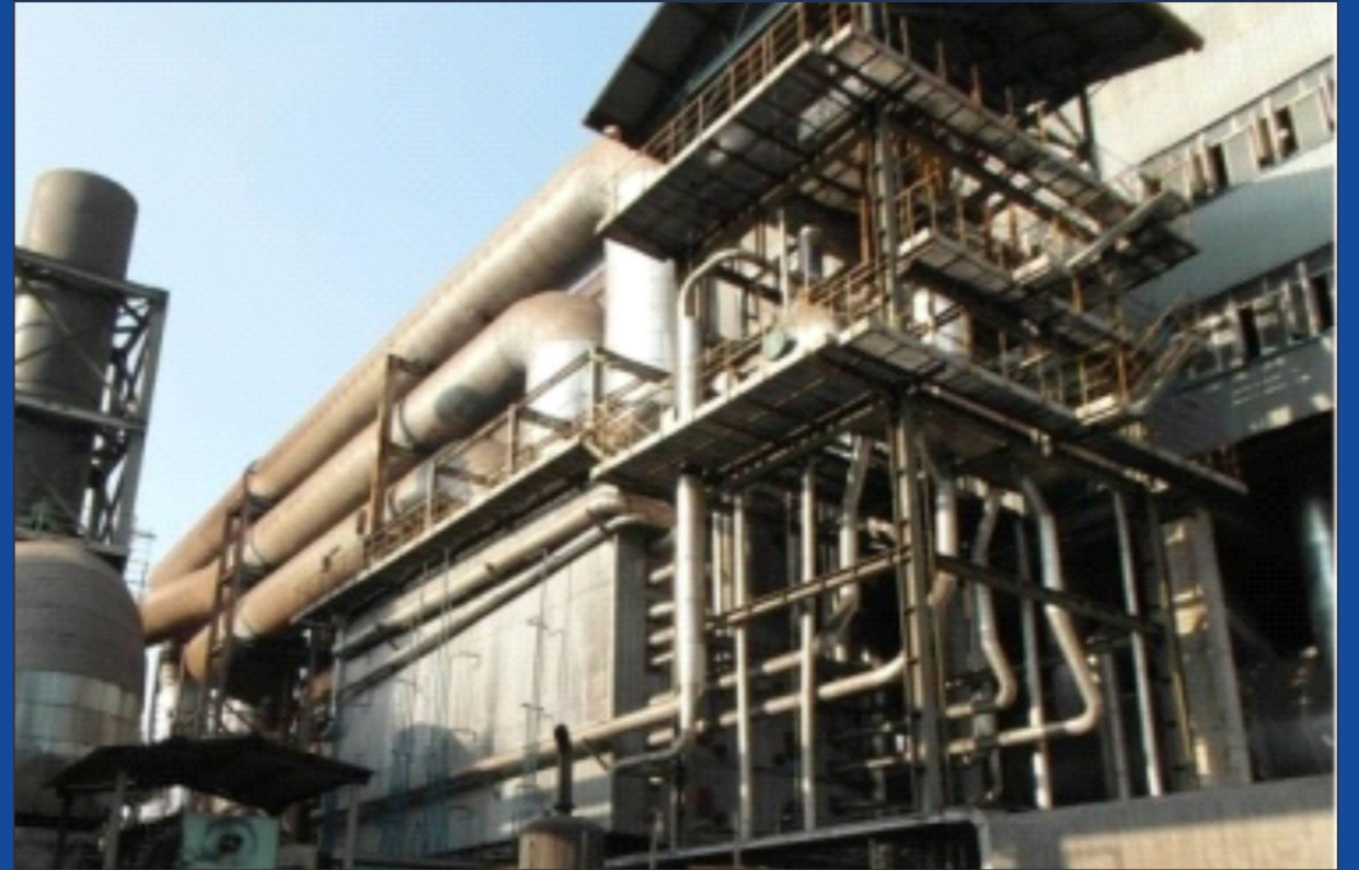
▼ Waste Heat Recovery Boiler for Sinterer (360m 2 ) in Weiyuan Steel
