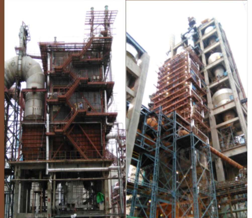
WHR Boilers for Raipur Line-1 6500TPD Cement Kiln Shree Cement Limited, India
