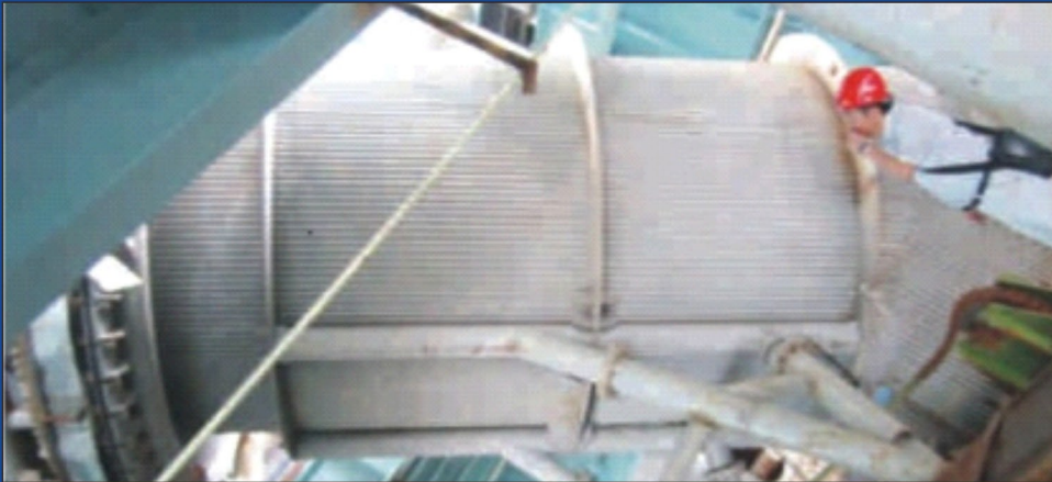
▼ Shaanxi Longgang 50t Converter Waste Heat Recovery Boiler
