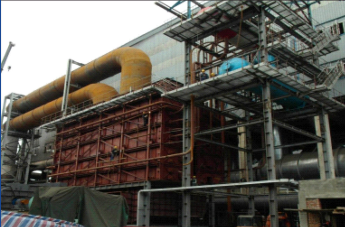
▼ Waste Heat Recovery Boiler for Sinterer (360m 2 ) in Weiyuan Steel
