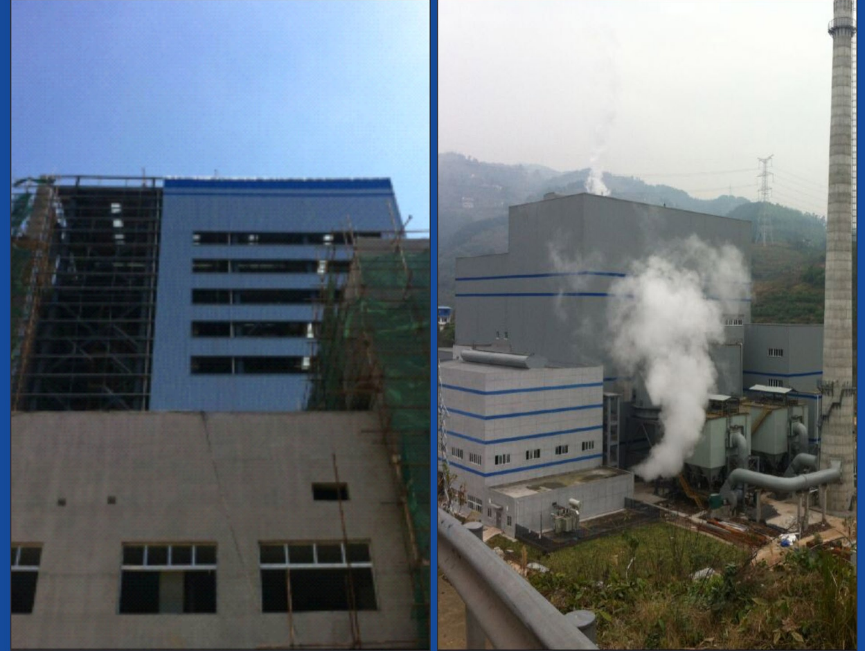
▼ 600 t/d Refuse Incineration Boiler in Xichang City
